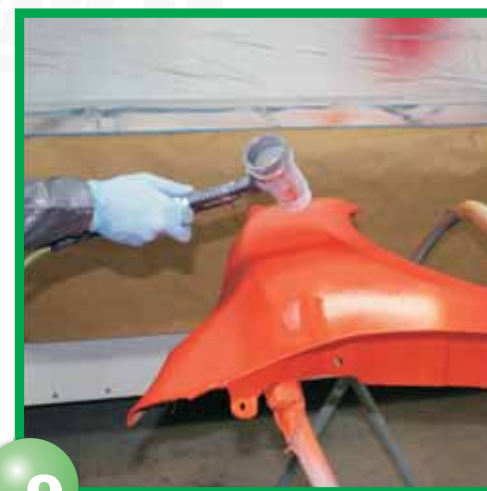
#15&16 Apply 2 to 3 medium wet coats of Auto Air Colors #4315. Allow coats to dry matte finish before re-coat, use waterborne dryer gun to assist dry time.
